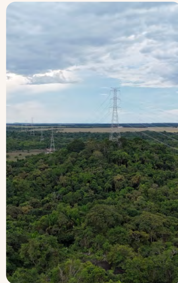
Transmission line- AXIA Collection
